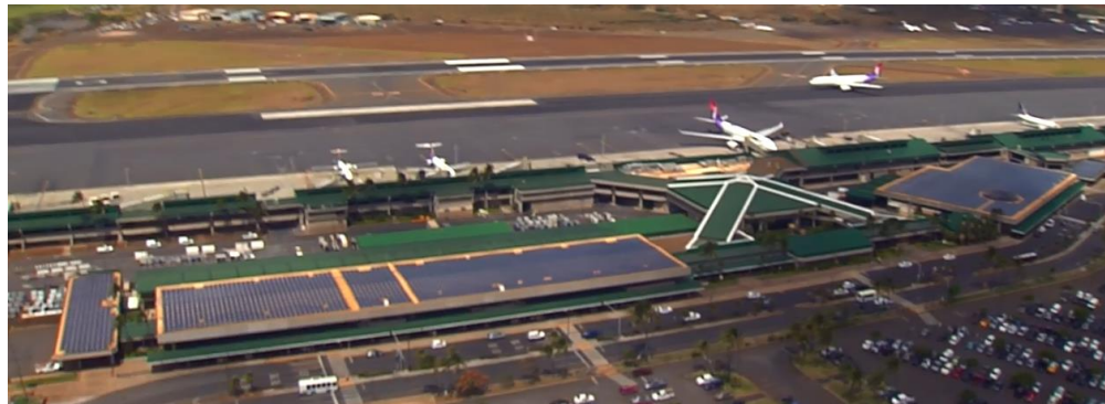
Kahului Ticketing and Baggage Claim Roof Installed 2015
